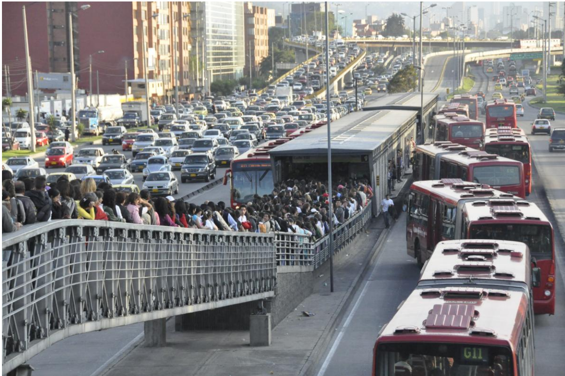
Figure 6 BRT TransMilenio in Bogotá
